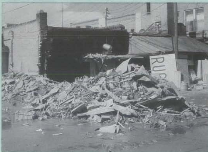
Damaged business after flood
